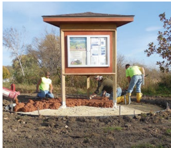
Building the kiosk at Erickson Conservation Area.
